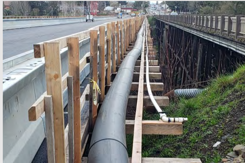
Temp pipe location needed to minimize wasted material and maximize protection from traffic.
