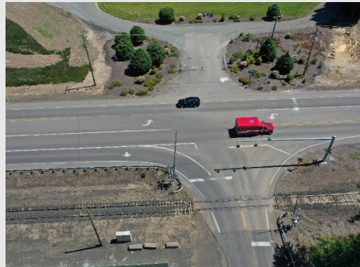
U.S. 20: Safety Upgrades, Albany to Corvallis
