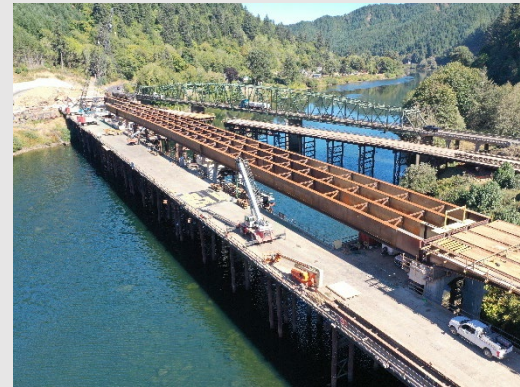
OR 38: Umpqua River (Scottsburg) Bridge Replacement
